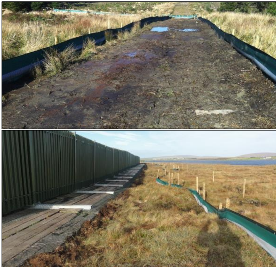
Plate 4-6 Silt Fence Details
