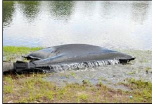
Plate 4-4 Silt bag under inspection
