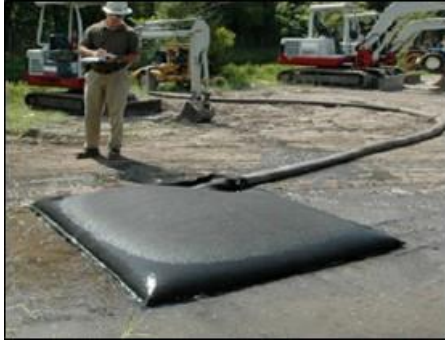
Plate 4-3 Silt Bag with water being pumped through
