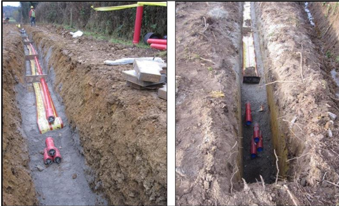
Plate 4-7 Typical Cable Trench View
