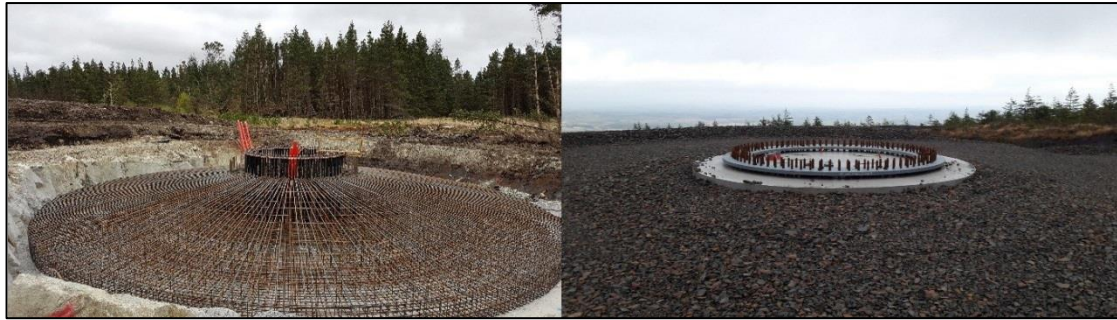
Plate 4-2 Turbine 'Anchor Cage' and finished turbine base
