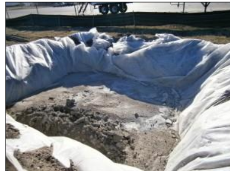
Plate 4-9 Concrete washout area
