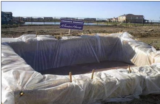
Plate 4-8 Concrete washout area
